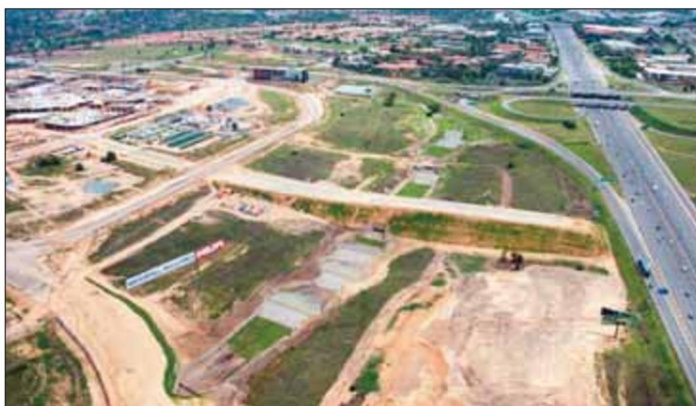
The location of the new overpass.
