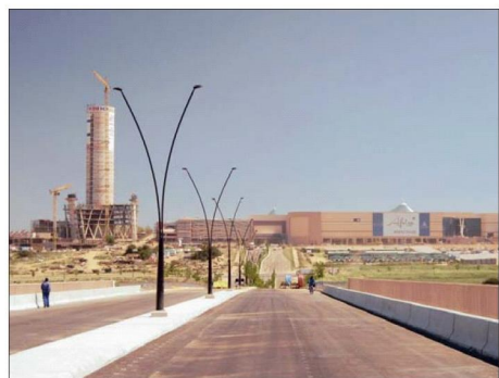
STUNNING: The Bridal Veil Road overpass bridge, developed by Atterbury Property Development, will open at the same time as Mall of Africa on Thursday.
